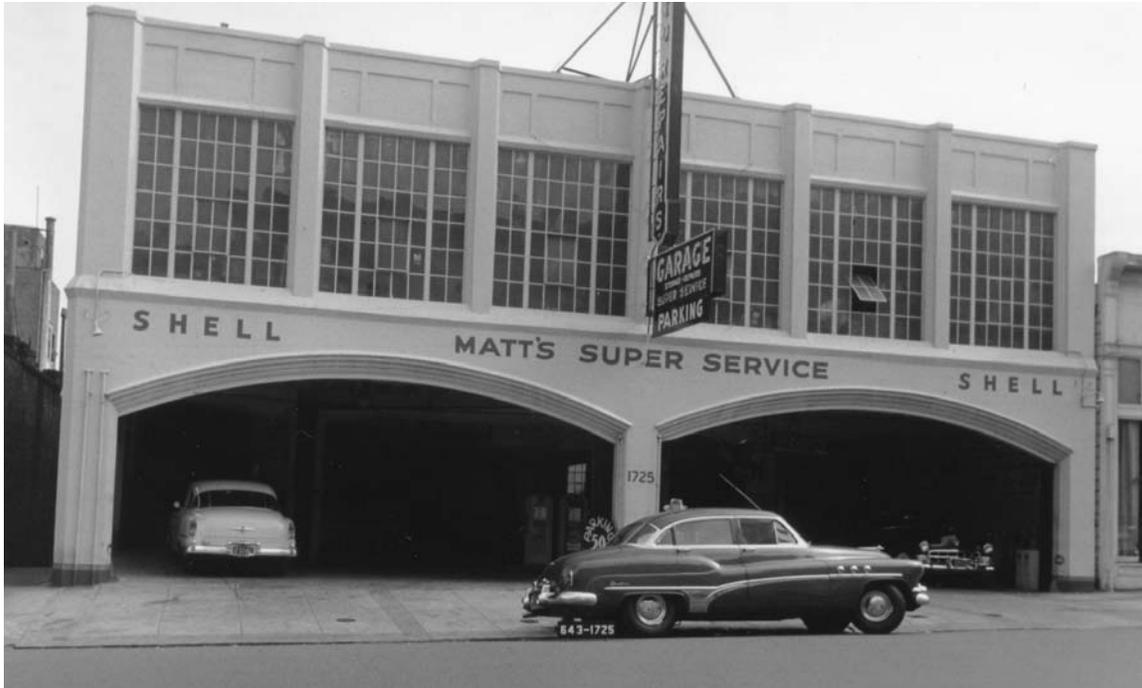
The Marius Bosc Garage, 1725 Sacramento Street, by architect Arthur S. Bugbee, 1923. This symmetrically-designed reinforced concrete garage still stands with all of its industrial steel sash windows intact. Photo: SFPL Assessor's negatives.
